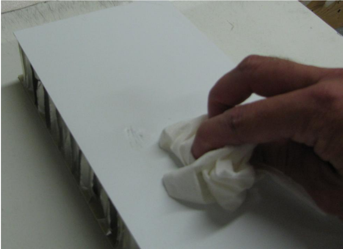
Figure 3: Clean area thoroughly with IPA
