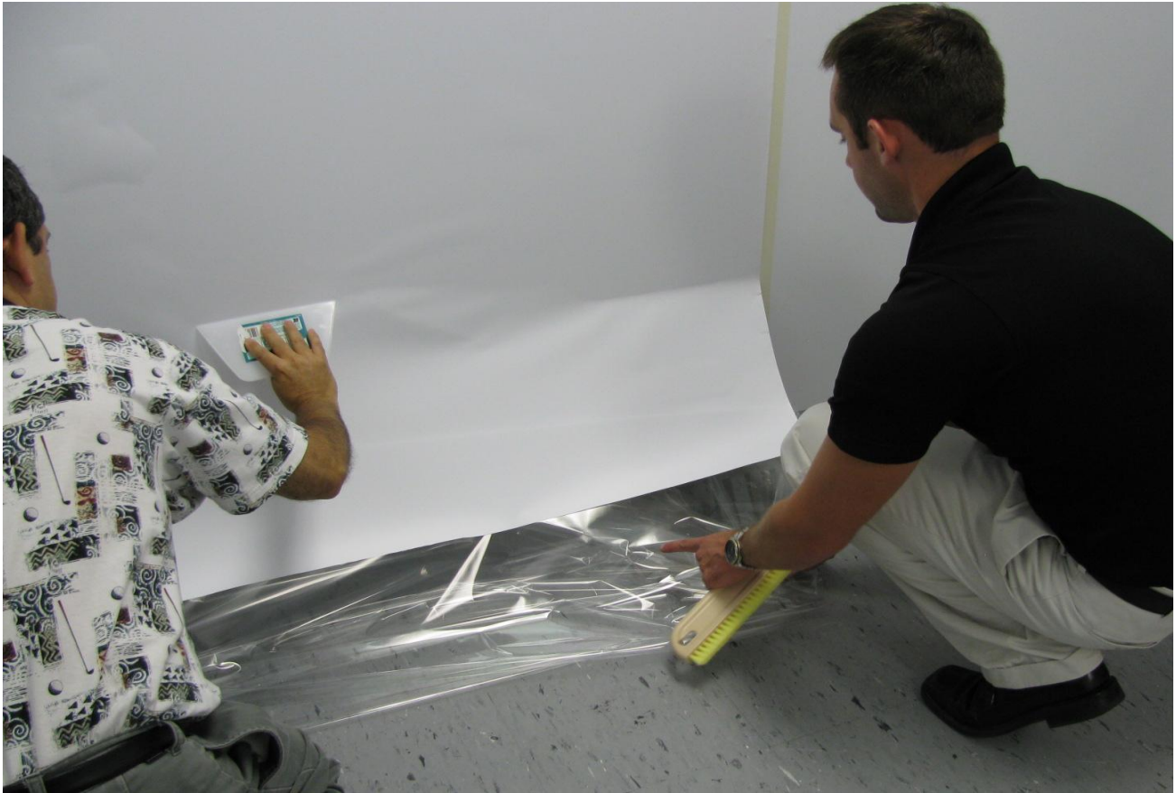
Figure 51: Keep clear backer film from bunching up under wall paper
