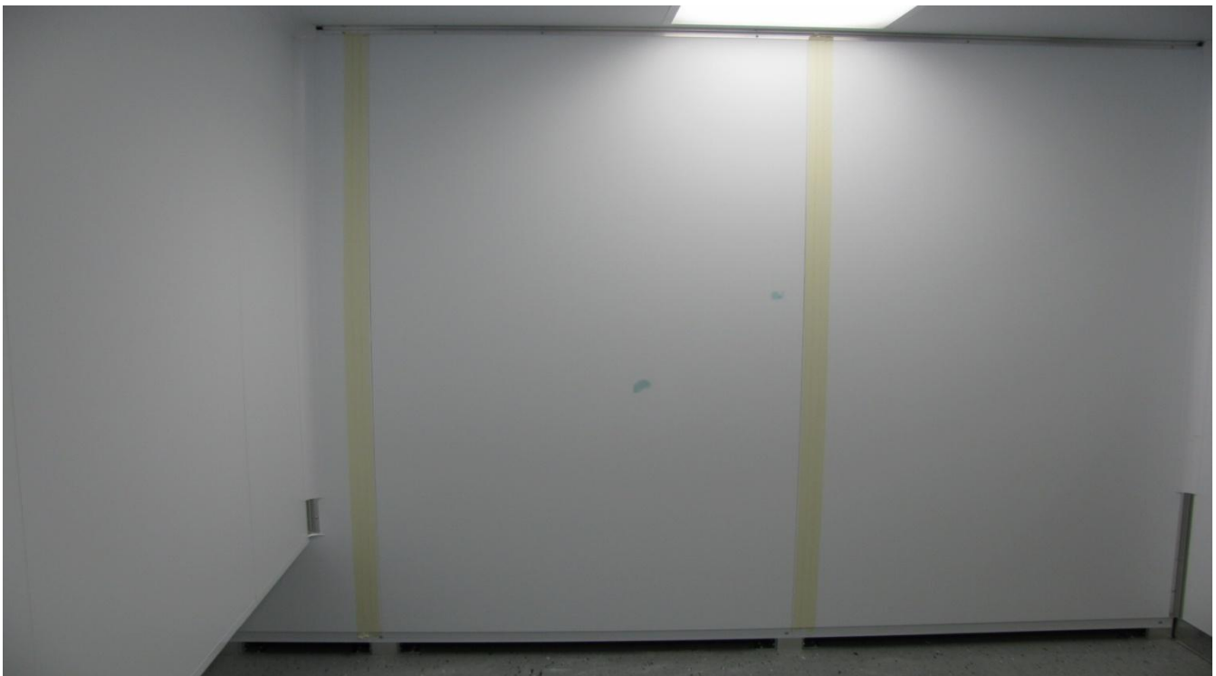
Figure 42: Tape off adjacent panels
