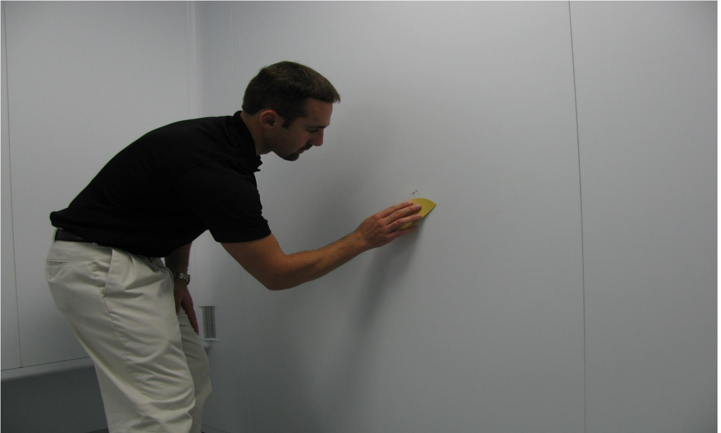
Figure 28: Sand the damaged area
