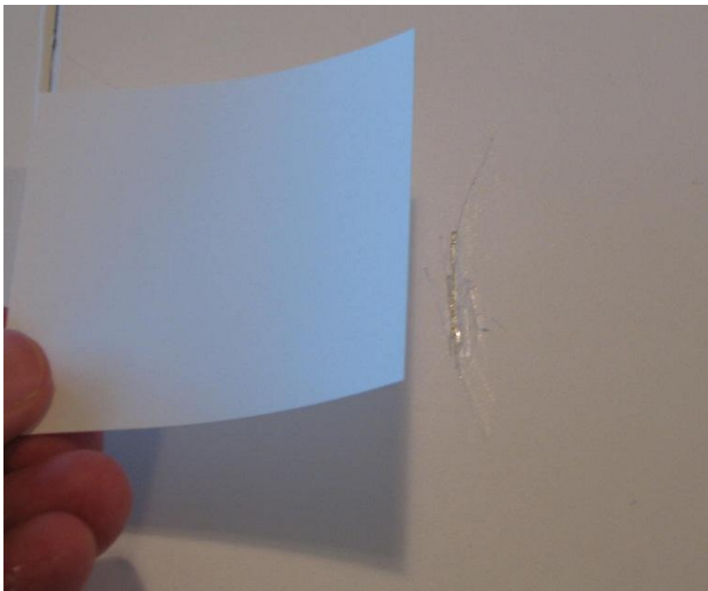
Figure 21: Be sure patch is sized to completely cover the damaged area
