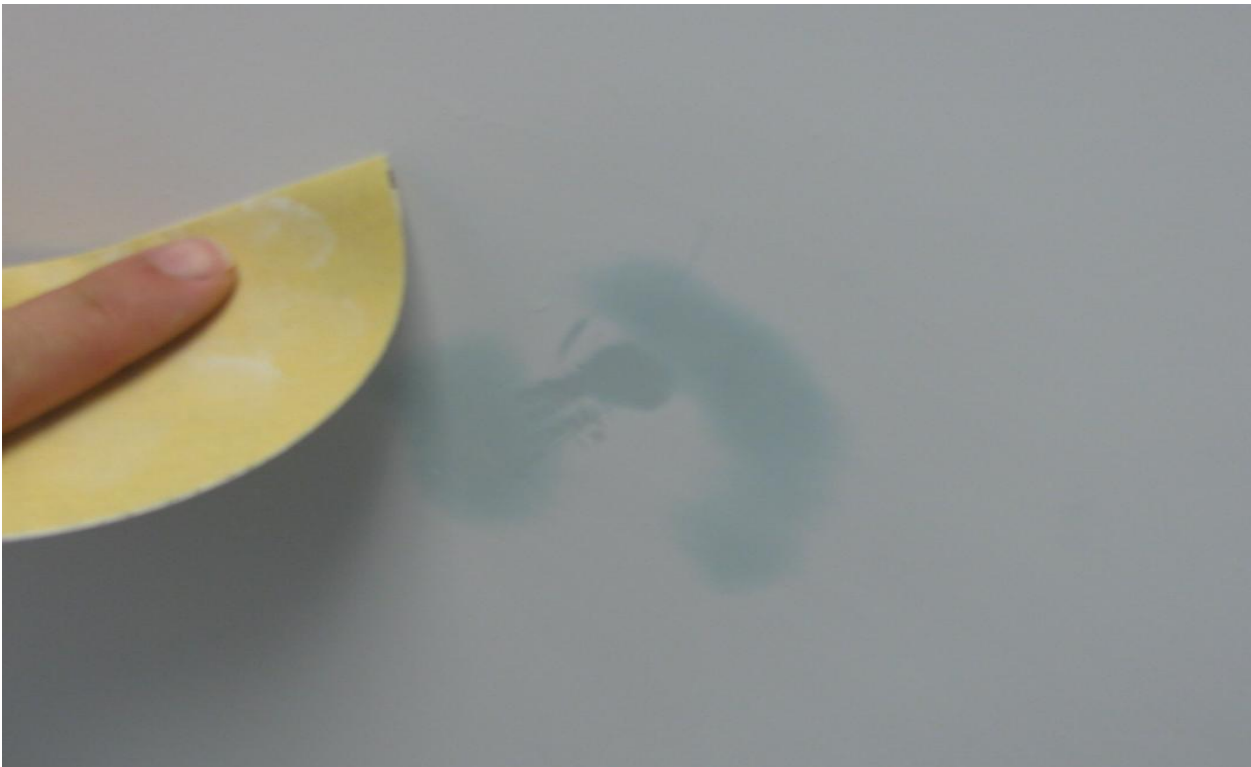
Figure 38: Close up of sanded filler material
