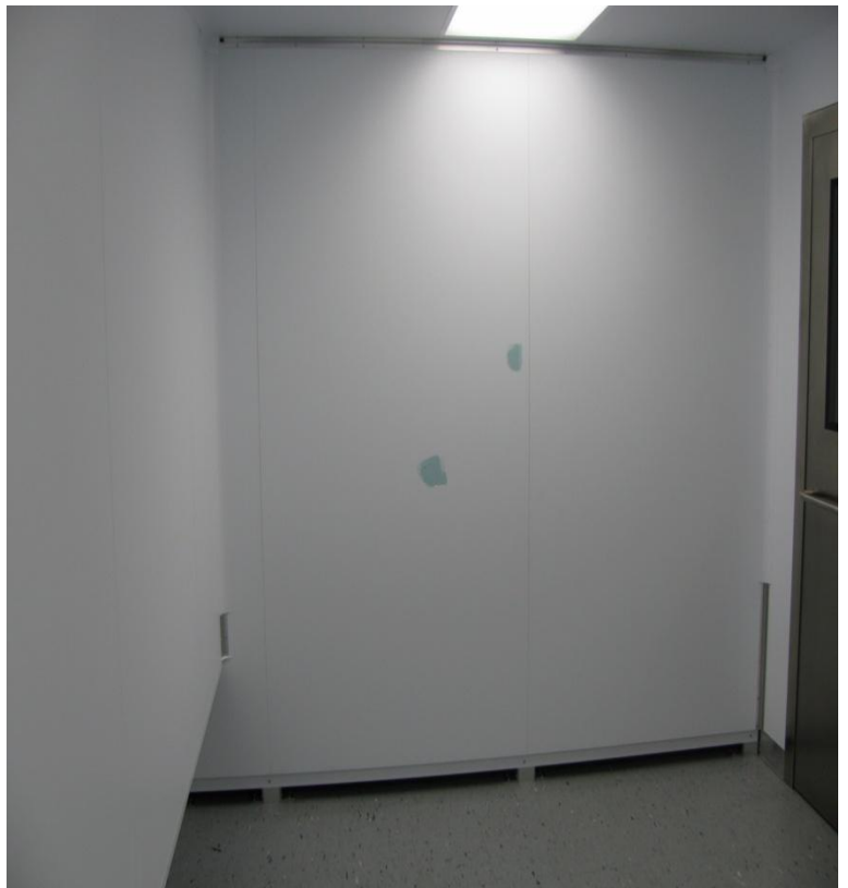
Figure 36: Panel with filler repair
