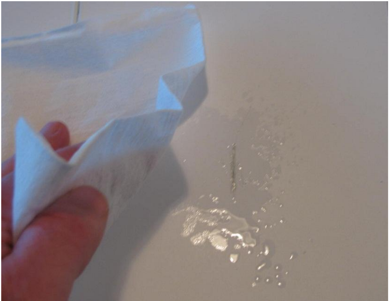
Figure 19: Thoroughly clean area where patch is to be applied
