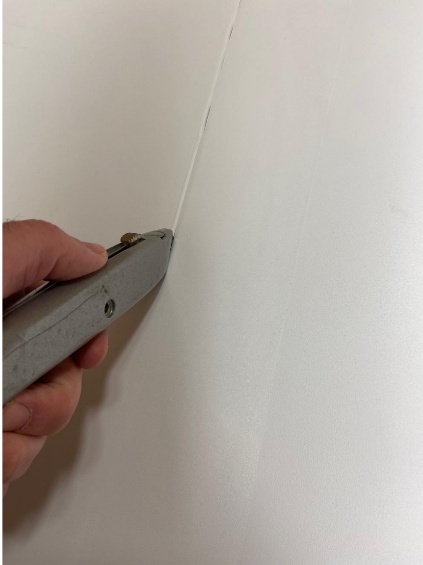
Figure 57: Use utility knife to trim vertical seams
