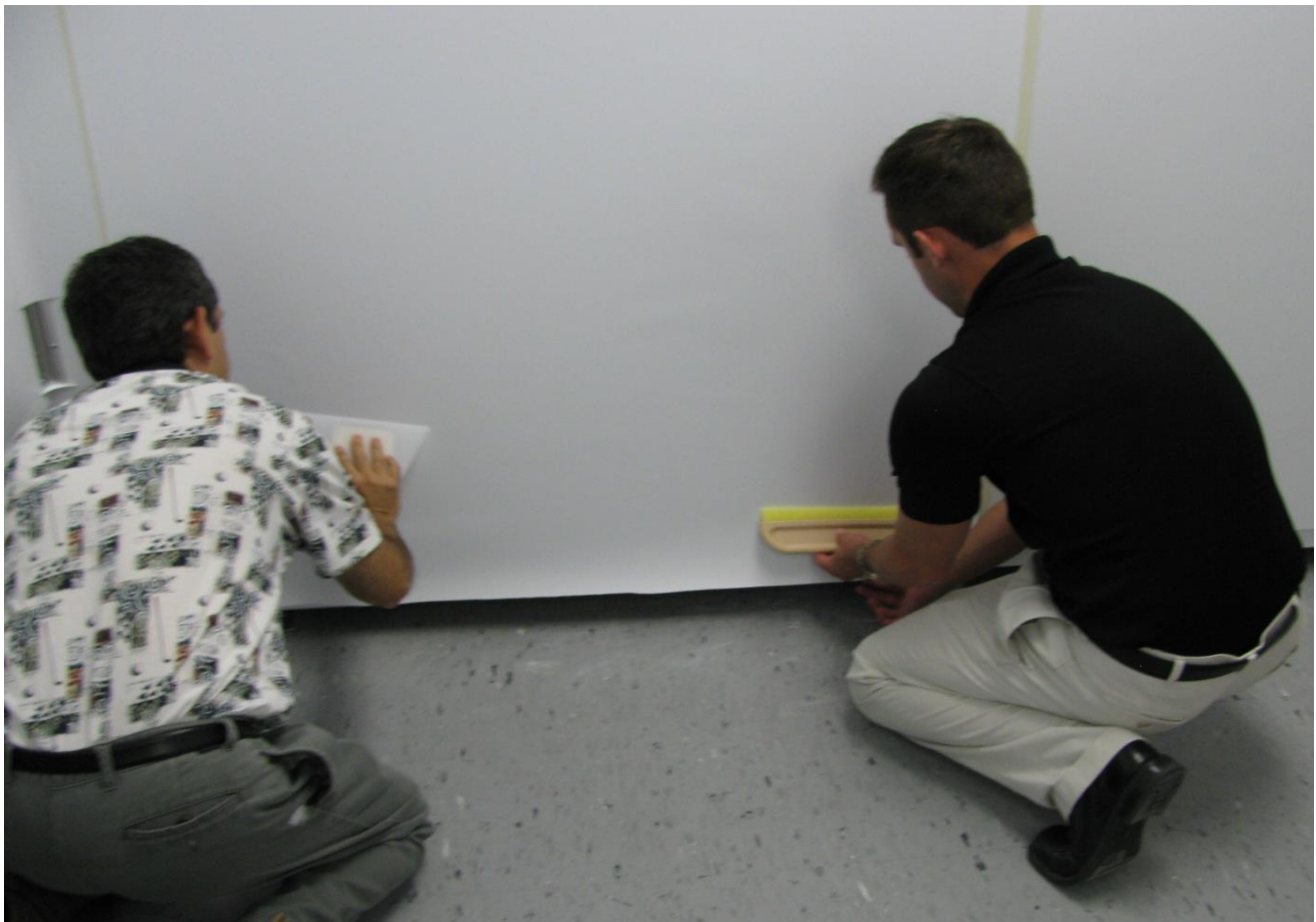
Figure 52: Remove backer film completely
