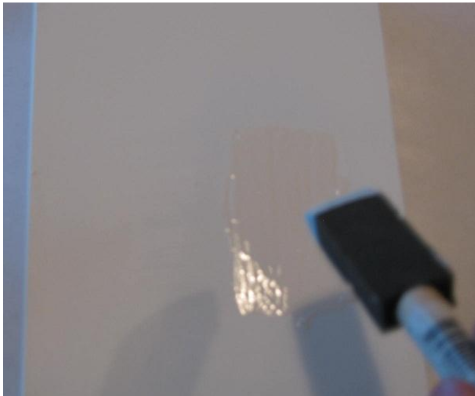
Figure 14: Blend in patch
