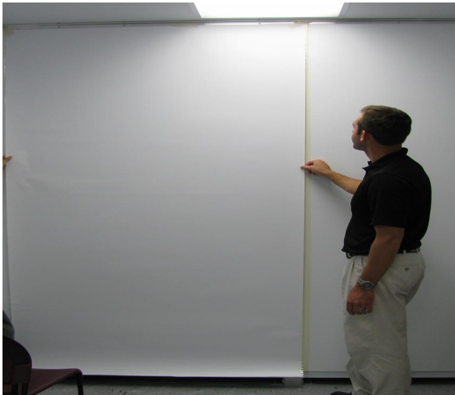
Figure 46: Allow wall paper to hang loosely
