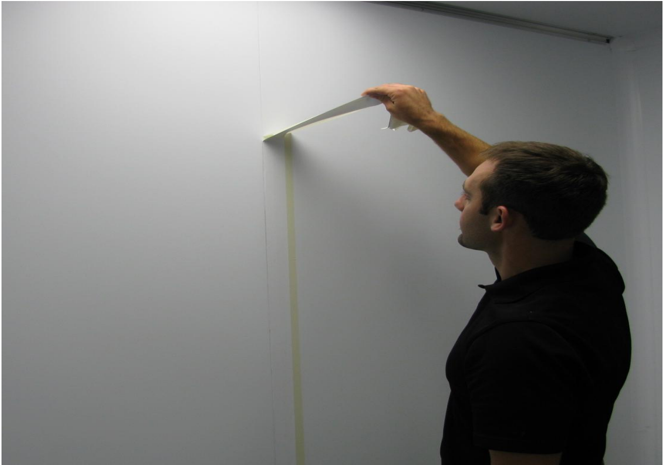
Figure 58: Remove tape and excess wall paper from edge
