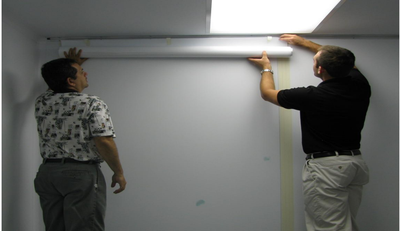
Figure 43: Tape uPVC wall paper roll in place
