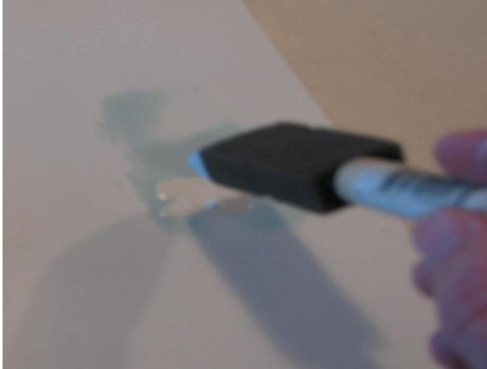
Figure 13: Apply paint to the damaged area
