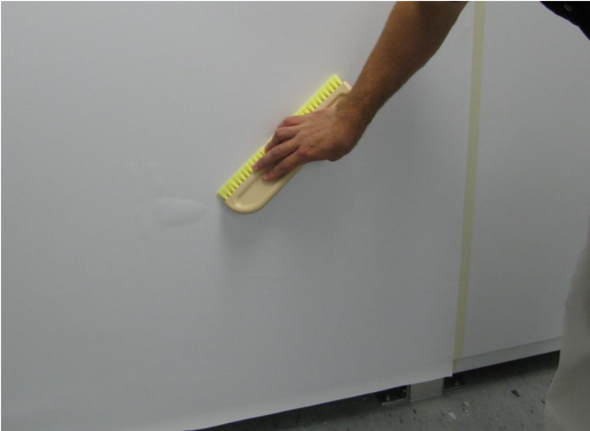
Figure 55: Wide straight edge will take out most bubbles
