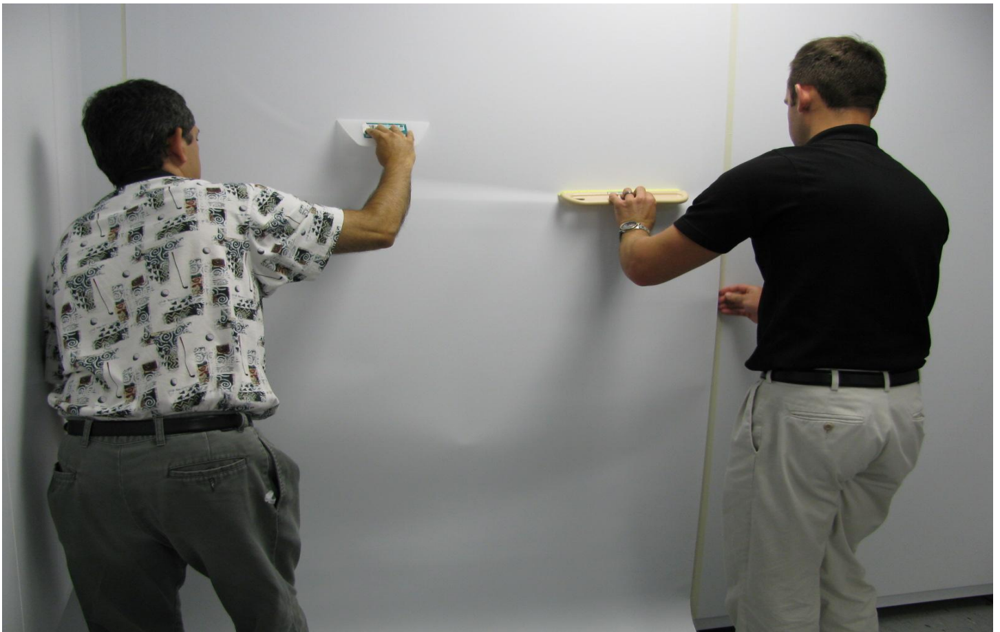
Figure 50: Smooth uPVC film as backer is removed
