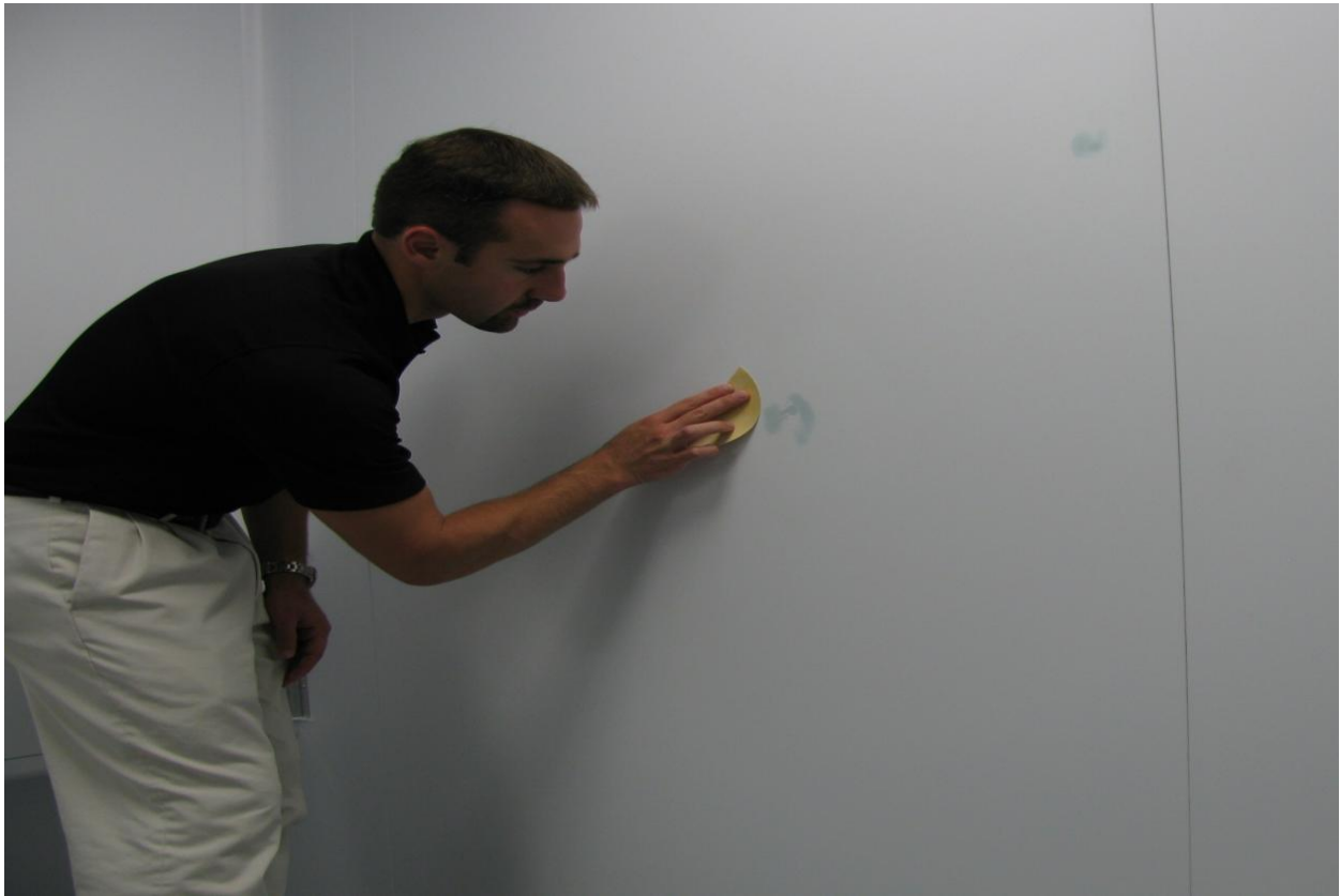
Figure 37: Sand filler material
