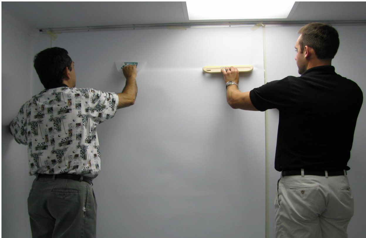
Figure 48: Smooth wall paper as clear backer film is removed
