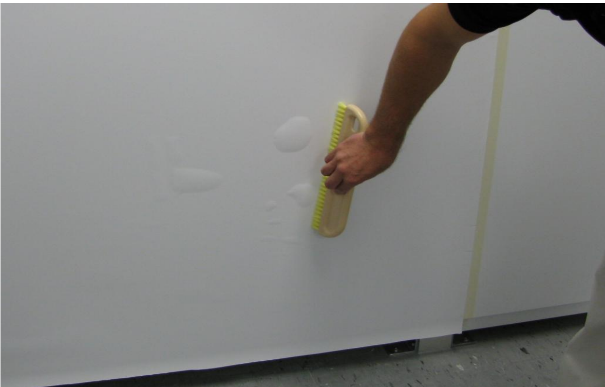
Figure 54: Start by smoothing over with wide straight edge or brush
