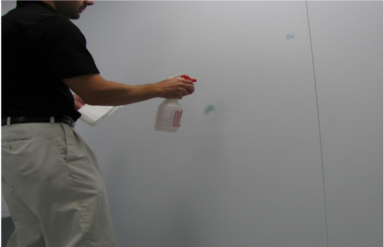
Figure 39: Spray down panel surface with IPA
