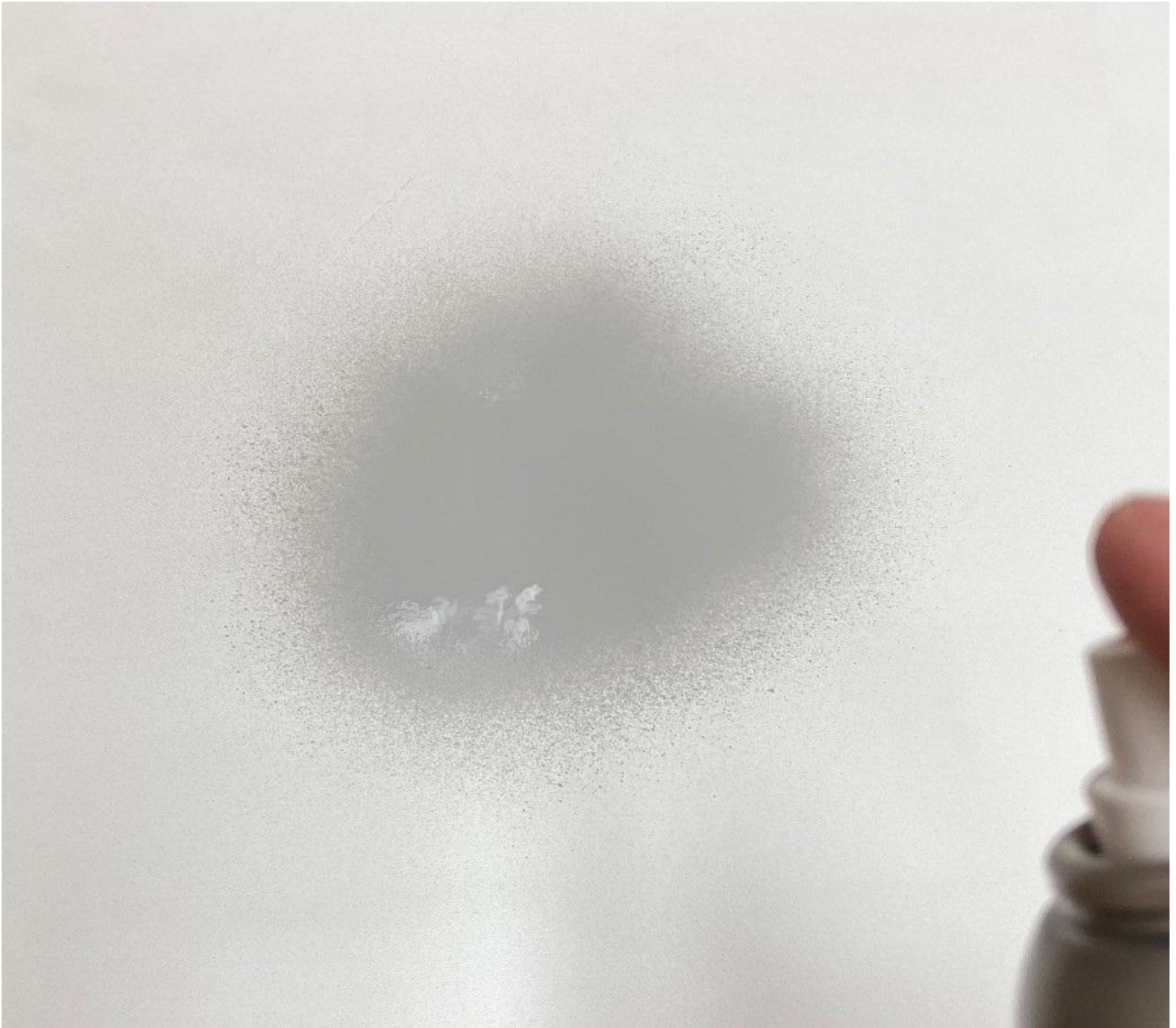
Figure 16: Apply primer coat
