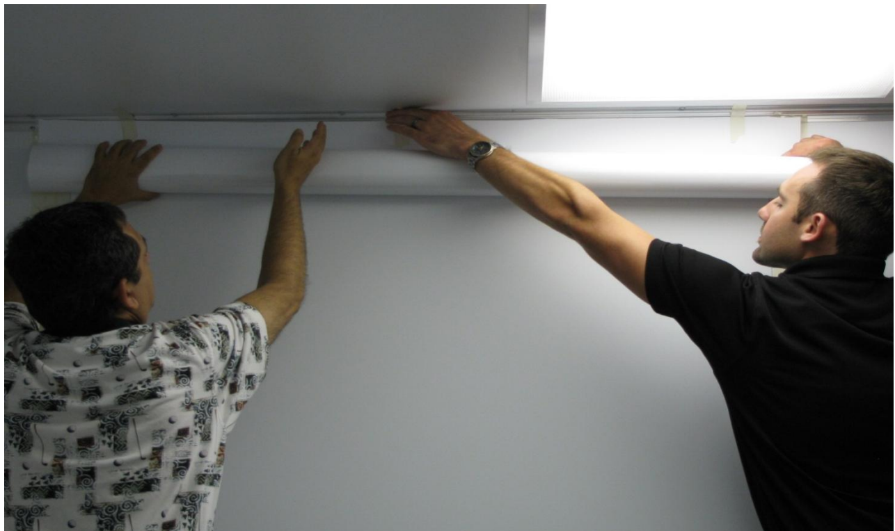
Figure 44: Tape uPVC wall paper roll in place
