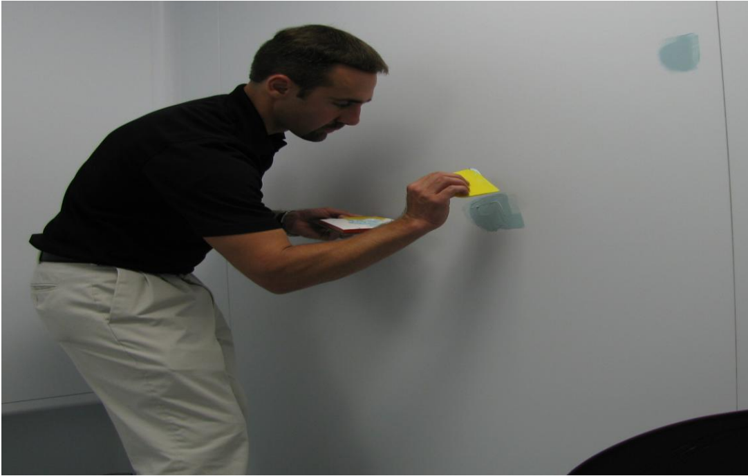
Figure 34: Apply filler material
