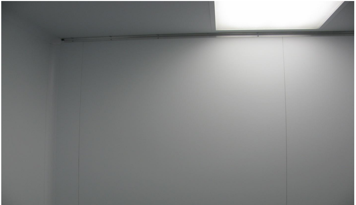
Figure 27: Coving removed above damaged panel
