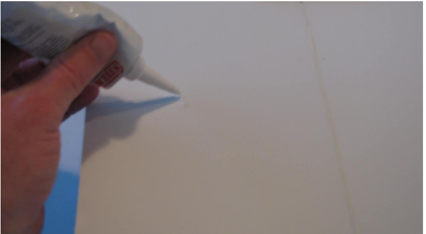
Figure 18: Apply cold weld adhesive bead to scratch
