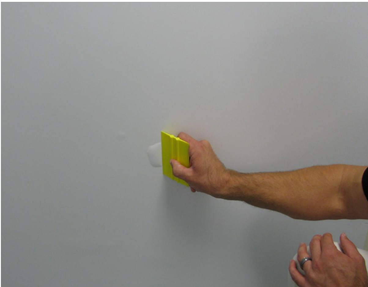
Figure 56: Smaller straight edge may be required for some bubbles
