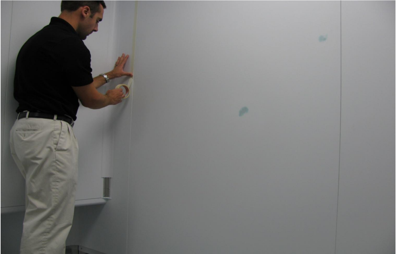
Figure 41: Tape off adjacent panels
