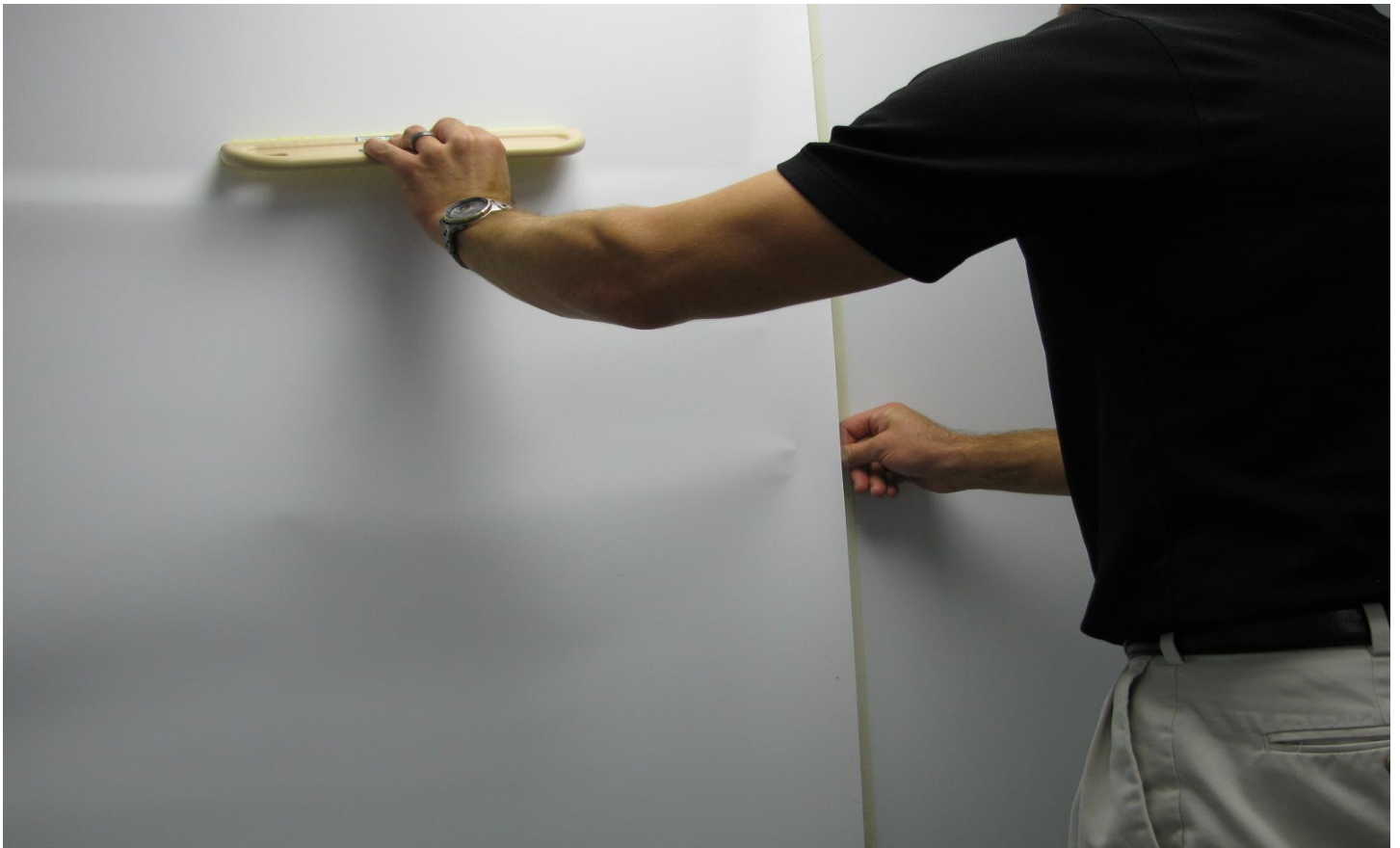
Figure 49: Removing clear backer film
